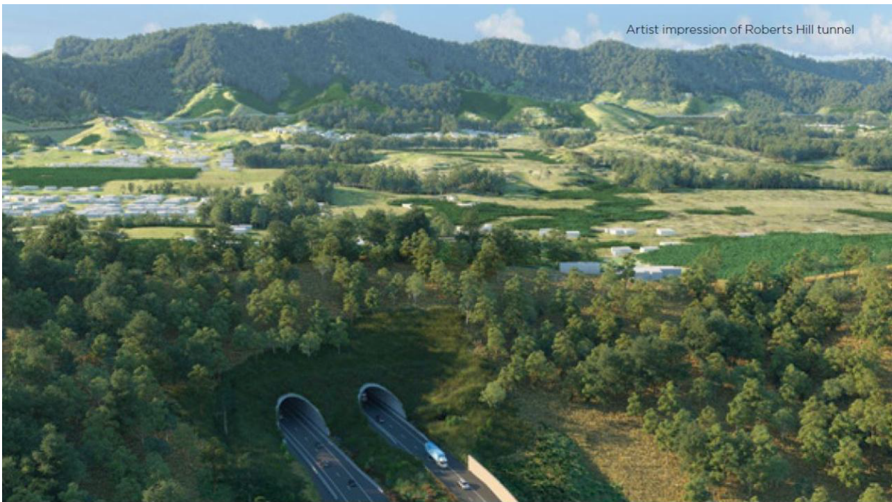
Three tunnels will be built on the Coffs Bypass for a combined length of just under a kilometre.
